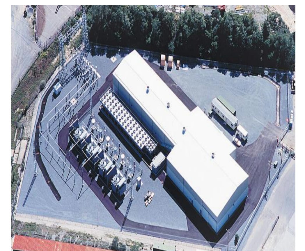
Onshore HVDC Converter
